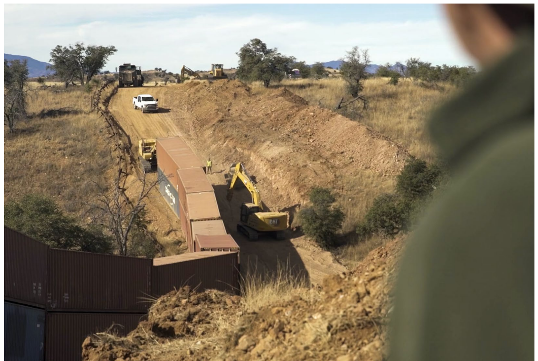
Arizona Gov. Doug Ducey’s illegal wall of shipping containers in the Coronado National Forest on Nov. 28, 2022. Screenshot: The Intercept/Kitra Cahana for The Intercept
